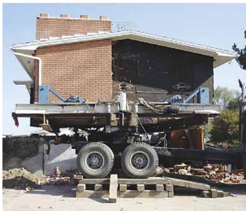
top: Kenny Pfeifer riding while in college above left: Western States Movers The Machine - engineered and manufactured by Kenny's Big Horn Machine Shop, The Machine enables them to keep a house perfectly level while moving over any terrain- courtesy of the family above right: Kenny bull riding at the Idaho High School Rodeo, Snake River Stampede arena - Gregg Photo
